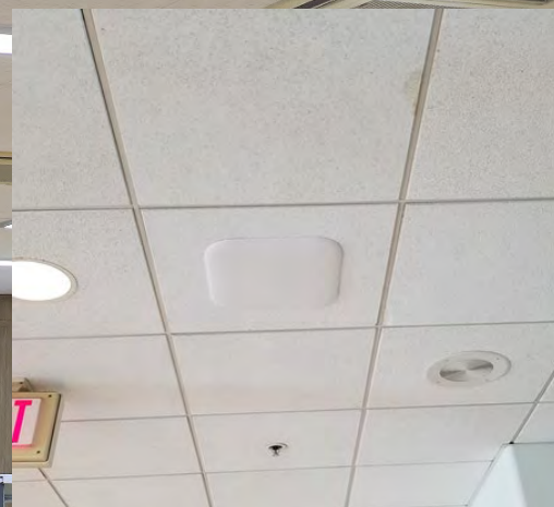
Oberon Envelop ™ Model 1040 recess mount for suspended and cloud ceilings conceals the AP behind a low-loss, low-profile plastic cover
